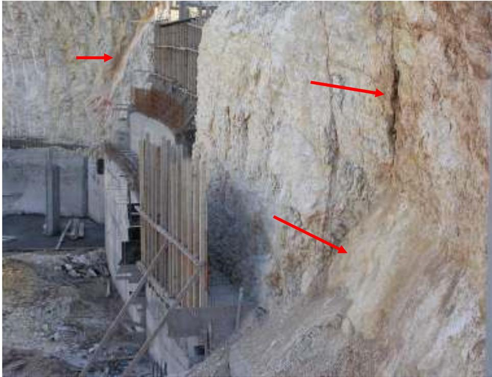
*Fig. 6 – Exposure of the Neshar fault plane in a foundation pit of a building in the junction between Oskar Shindler road and Mendel Zinger St.*
